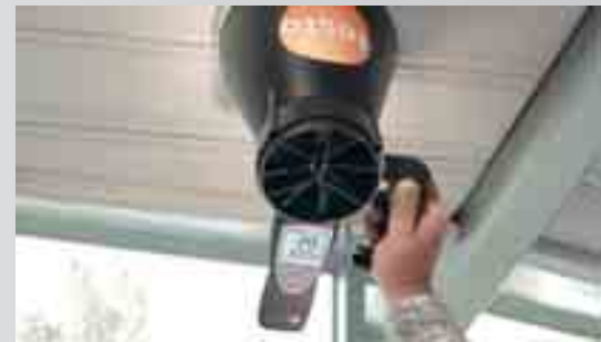
Monitoring ingoing air in a disc outlet
