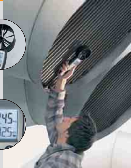
Volume flow measurement with a large Ø 100 mm vane at duct outlet
