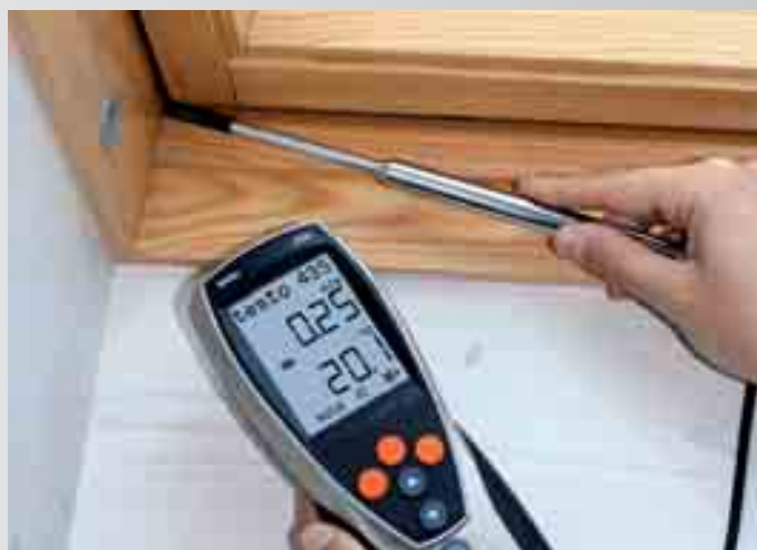
Measuring flow at a leaking window
