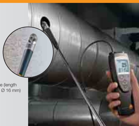
Monitoring air velocity in air conditioning ducts
