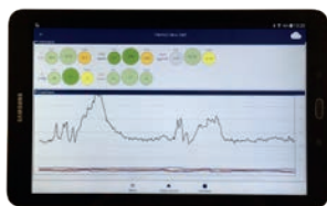
Wall-mounted tablet for displaying live data
